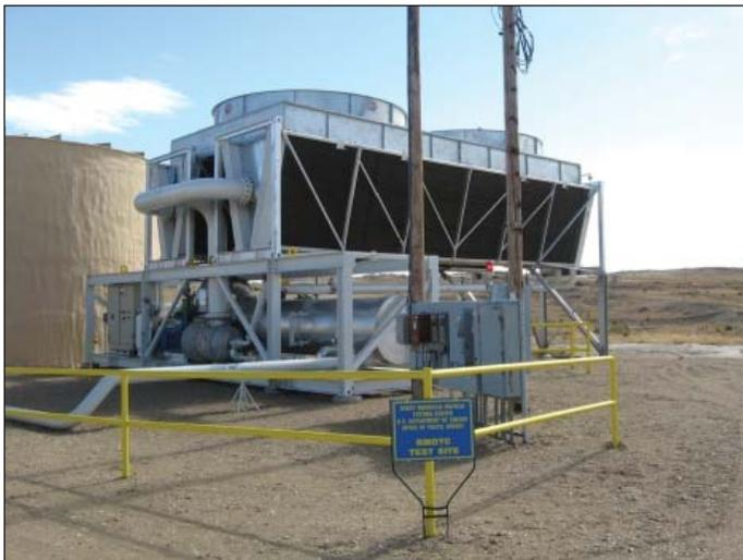
**Figure 4.** Organic Rankine Cycle (ORC) 250 kW low-temperature geothermal system at NPR-3.
